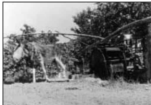
Old methods of pumping water
