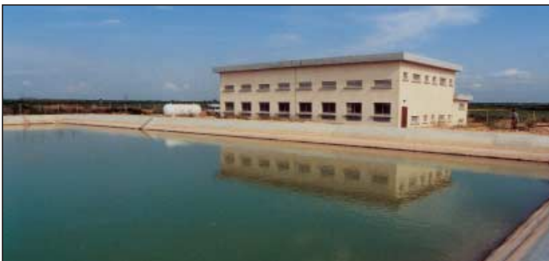
Central Distribution Point at Kokkinokhoria
